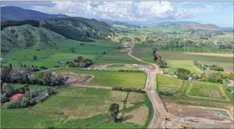
The haul road built near North Manakau Road. Photo: NZTA
